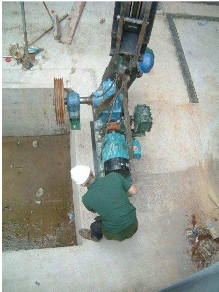
Left – positioning the winding gear.
