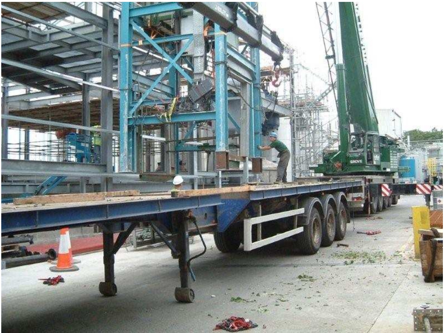
Above – the new feet are secured to the lift base.
